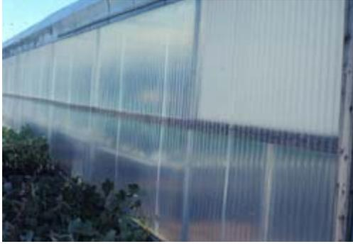
**Fiberglass** was widely used in the 1960's and 1970's. Its use has declined significantly due to newer materials such as the polycarbonates and acrylics being made available. Fiberglass has a tendency to discolor after about 8-10 years reducing light transmission greatly. It also burns very easily and has no great insulation value.
